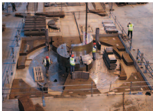
Construction of the Second Target Station shield monolith.
