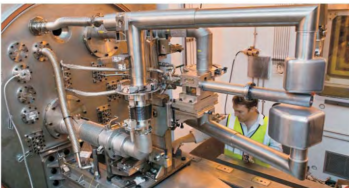
► Robin Burrigde (ISIS) inspecting a newly-installed cabinet of radiation monitors for TS-1's services area. The monitor heads are positioned around the services trolley to detect any changes in background levels and to highlight any fluctuations within the \text{D}_2\text{O} water cooling circuits during operation. 09EC2045
