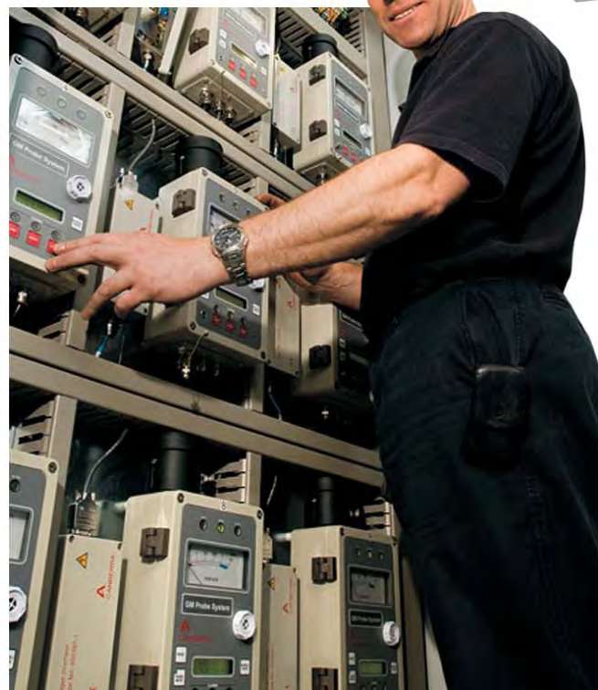
► Robin Burrigde (ISIS) inspecting a newly-installed cabinet of radiation monitors for TS-1's services area. The monitor heads are positioned around the services trolley to detect any changes in background levels and to highlight any fluctuations within the \text{D}_2\text{O} water cooling circuits during operation. 09EC2045
