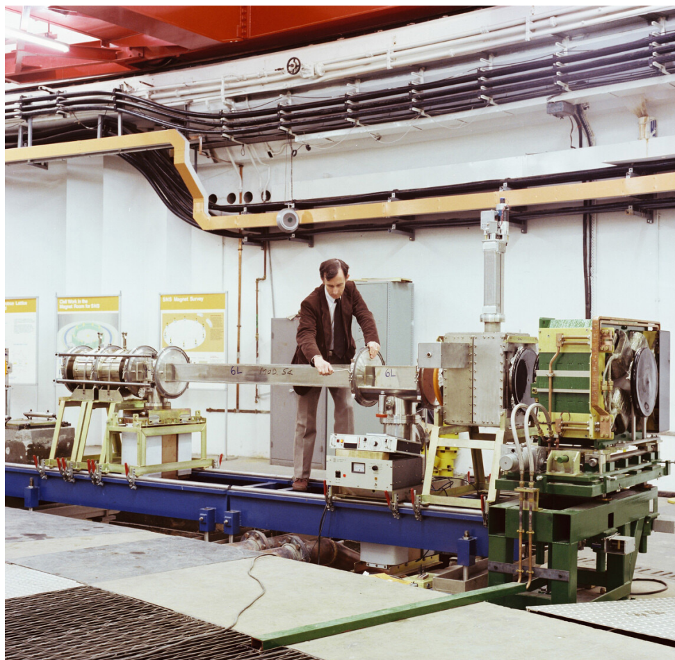
Peter Parry assembling part of the vacuum system during synchrotron build progress, June 1983.
