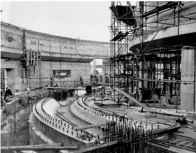
The Nimrod accelerator being installed into the synchrotron hall. Nimrod was a 7 GeV proton synchrotron for particle physics experiments.
