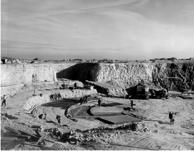
Excavation for the foundations of the Nimrod synchrotron, which operated at the Rutherford High Energy Laboratory between 1964 and 1978.
