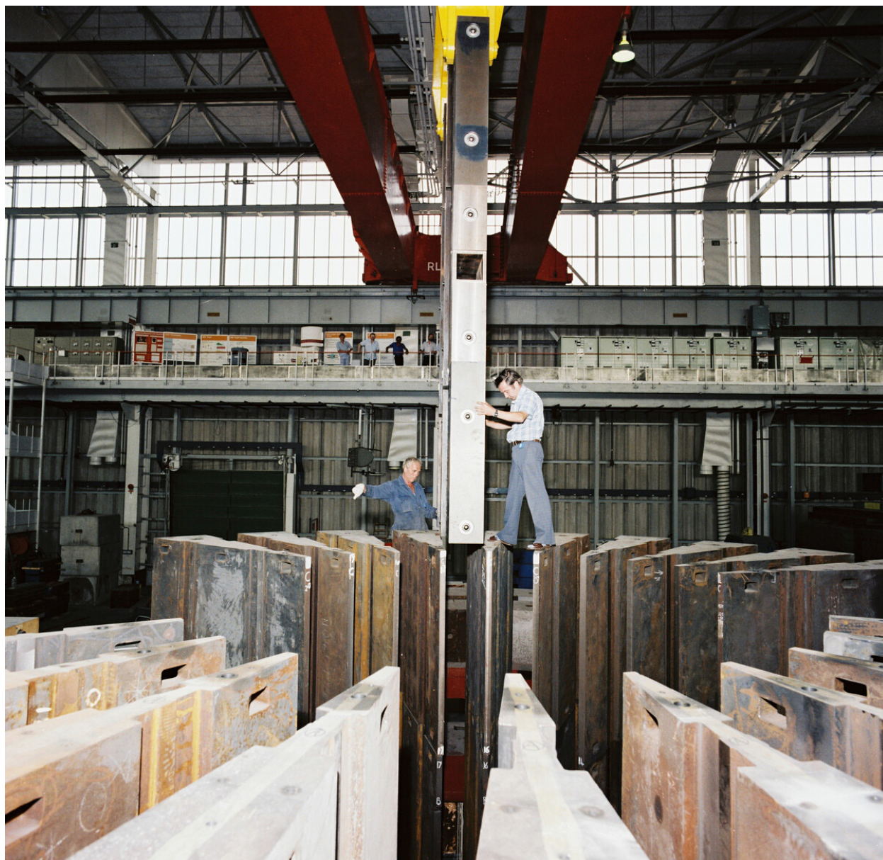
Brian Culley and Colin Thomas check that a shutter assembly will fit during neutron beam shutter installation in 1983. Personal protective equipment and working from heights were less regulated in the early construction.
