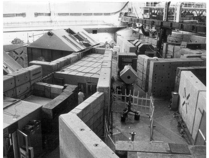
The Nimrod accelerator being installed into the synchrotron hall. Nimrod was a 7 GeV proton synchrotron for particle physics experiments.
